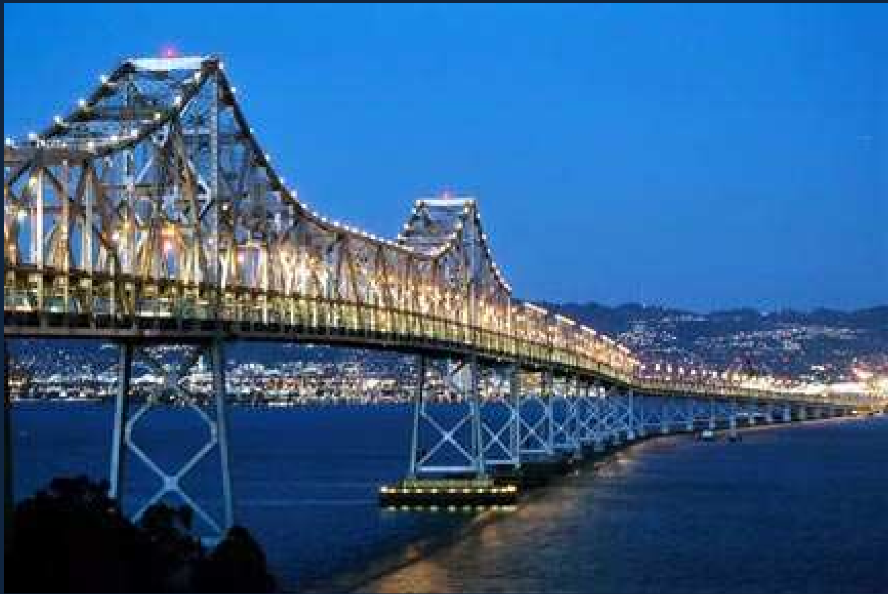
Le pont East Bay San Francisco
